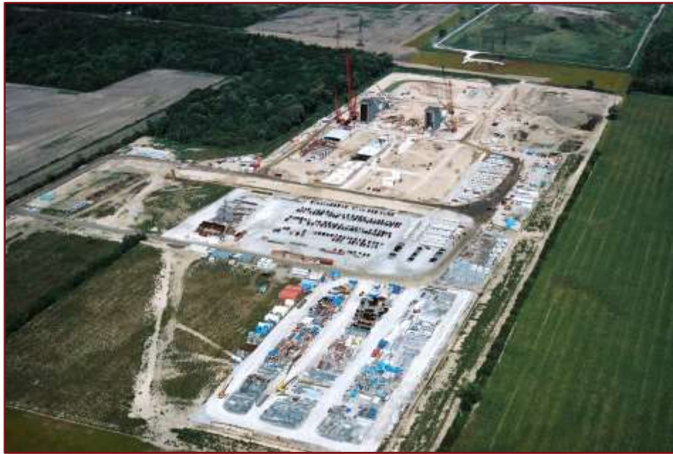
Image 2: Oblique Aerial Photograph of Project Area, Dated May 14, 2008
